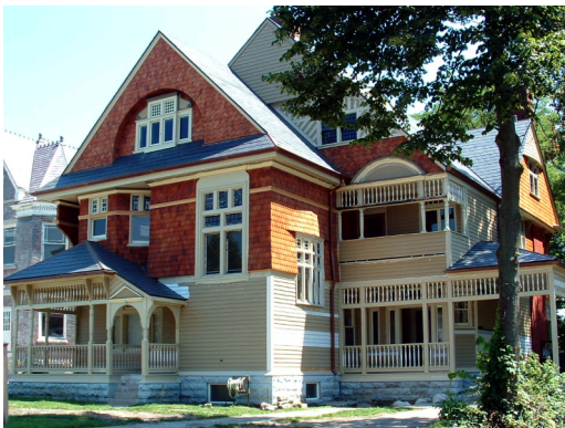
The varied decorative wood patterns found on the Dimond House (currently under restoration) are a distinctive Queen Anne feature, although the dominance of wood shingles places it as a Shingle Style house as well.
