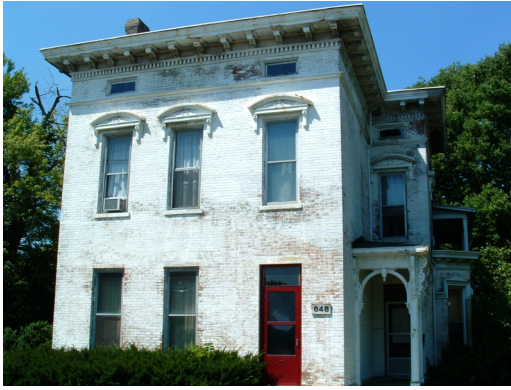
The Weimer House at 648 East High Street displays most of the classic features of an Italianate house.
