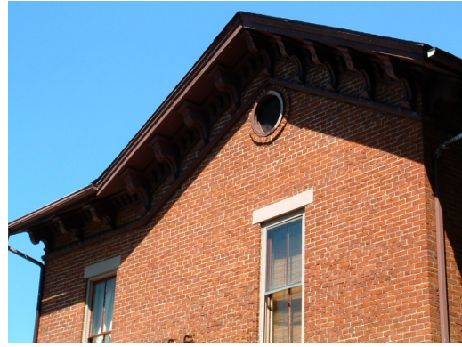
Two-over-two windows and bracketed cornices on a neighboring house farther down East High.
